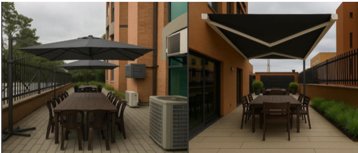
Figure 73: Terrace Renovation and Optimization
