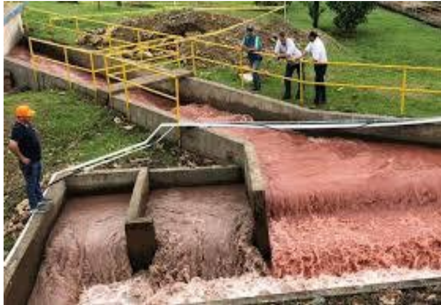
Figure 66. Modernization of the La Esmeralda Drinking Water Treatment Plant (DWTP)
