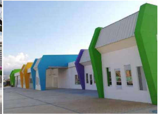
Colegio Torrente – Soacha,
